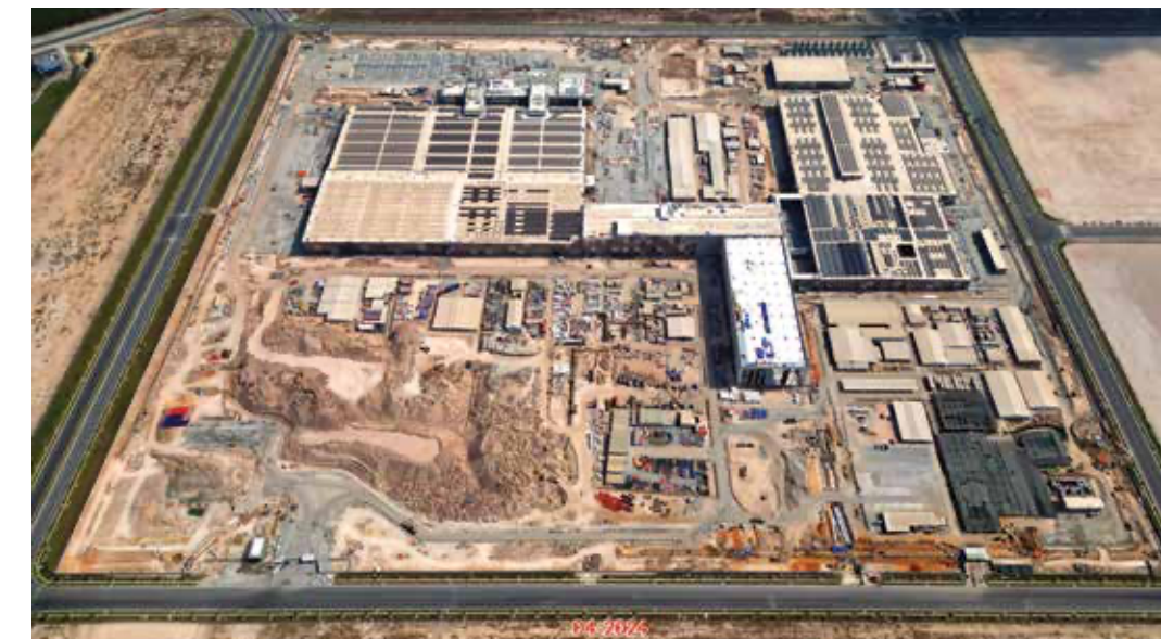
Panoramic view of jobsite execution.
