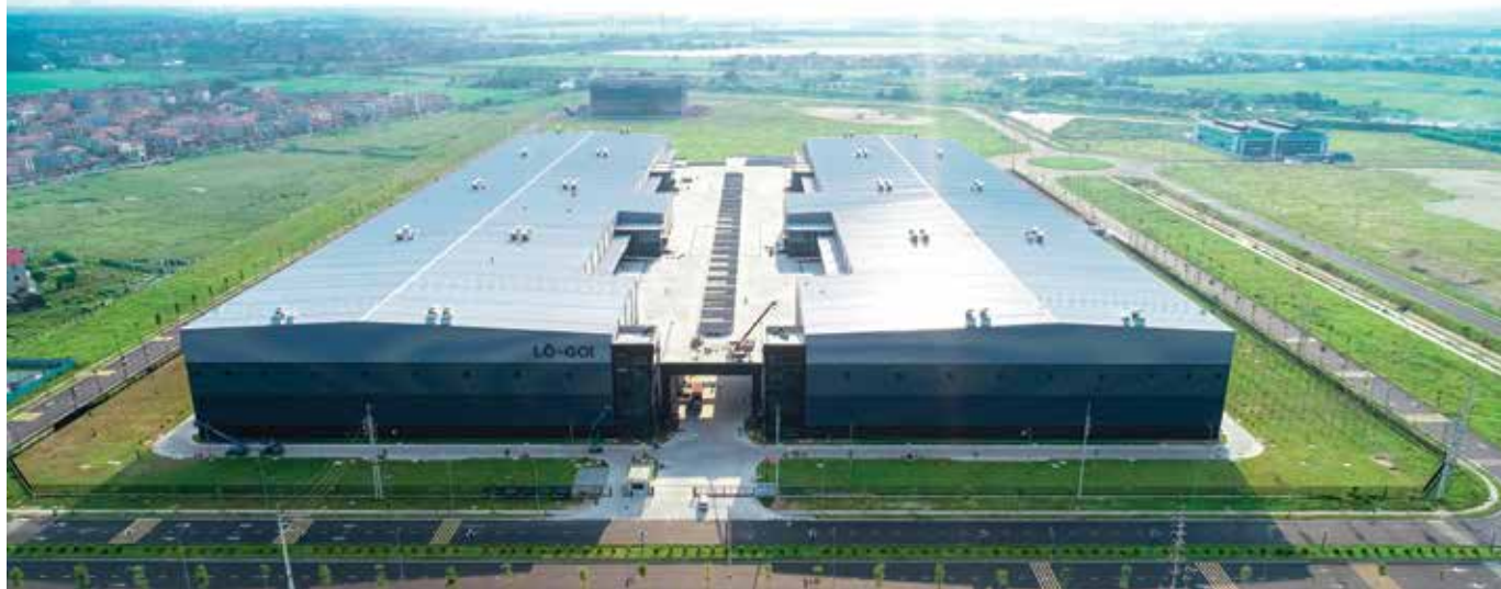
At Yen Phong II-A Industrial Park (Bac Ninh), Cotecons and LOGOS Property Group have created a brand-new two-storey Industrial & Logistics Complex in Northern Vietnam, built to LEED Gold green standards, pioneering the trend toward modern, automated, and sustainable logistics.
