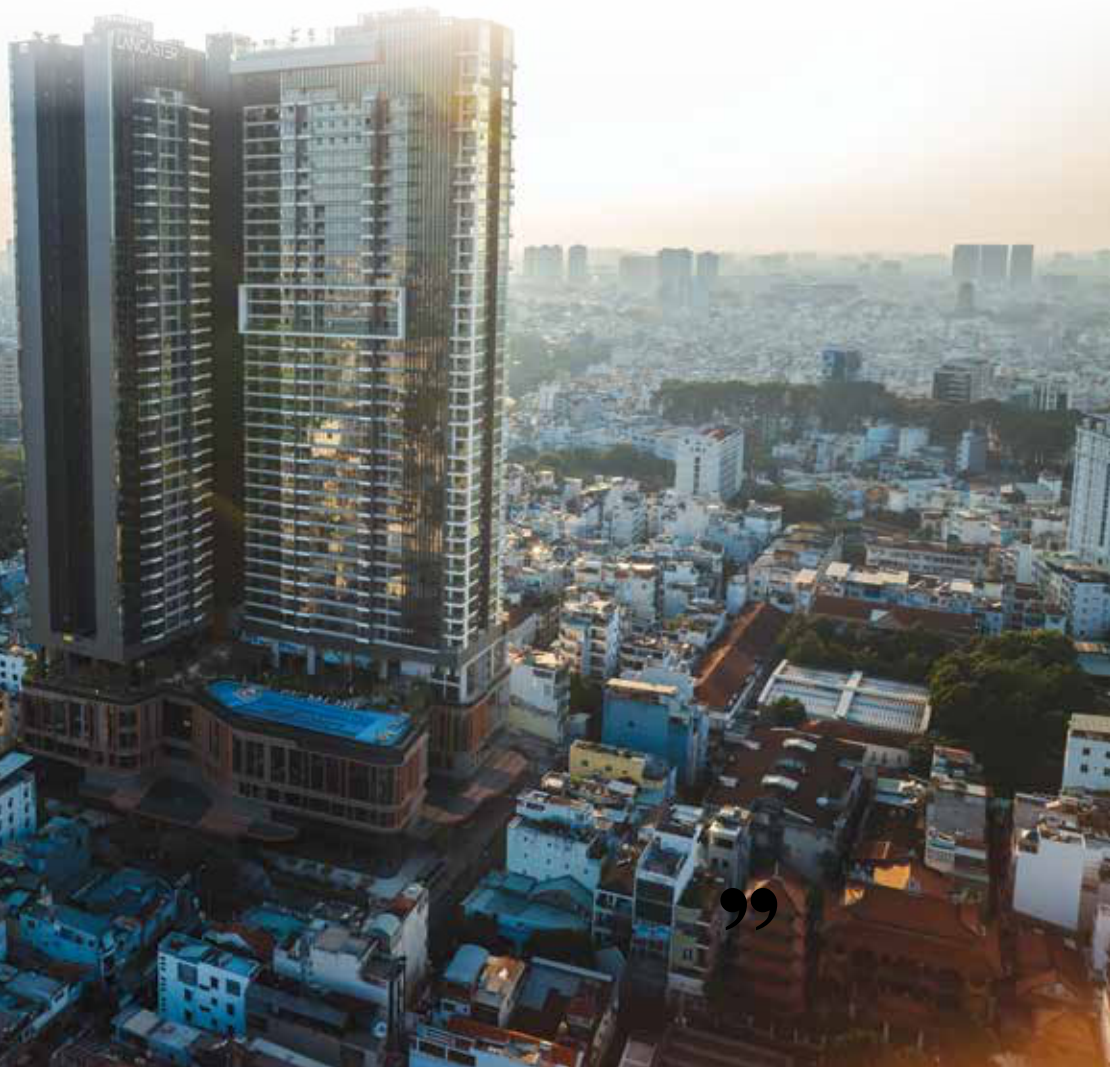
Overview of the Lancaster Legacy project (HCMC) - a collaborative venture between Coteccons and Sinh Nam Façade.
