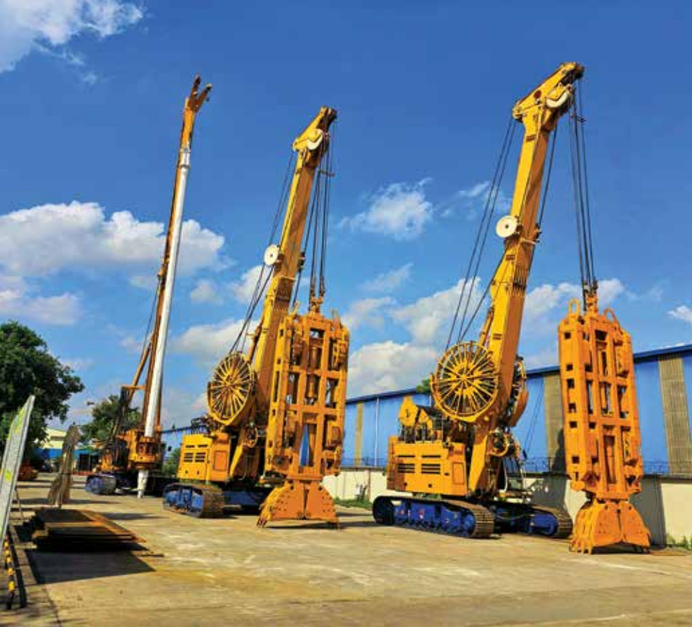
GEO Foundations' heavy equipment array deployed at the Binh Duong depot (HCMC).
